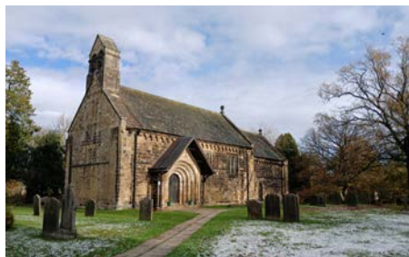
Adel Church, north Leeds (12th century).
